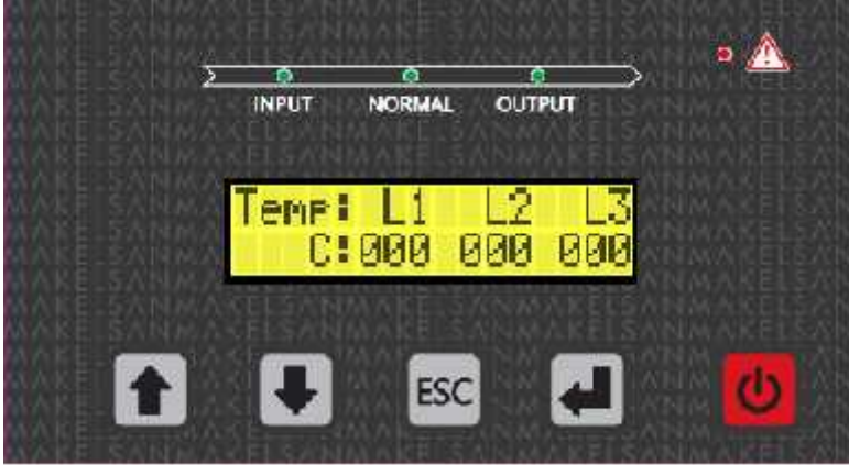
) Transformer Temperature Information (L1,L2,L3)
